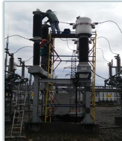
La construction de la sous-station 155 "Bolchekamenskaya" "PAO Tatneft"
